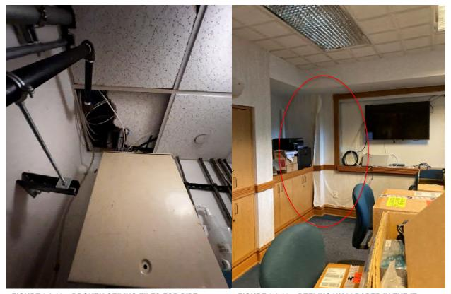
FIGURE 2.3.08 – BROKEN CEILING TILES FOR PIPE PENETRATIONS.
