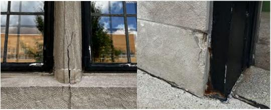
IMAGES 3.1.07 LIMESTONE CRACKS AND CHIPS
