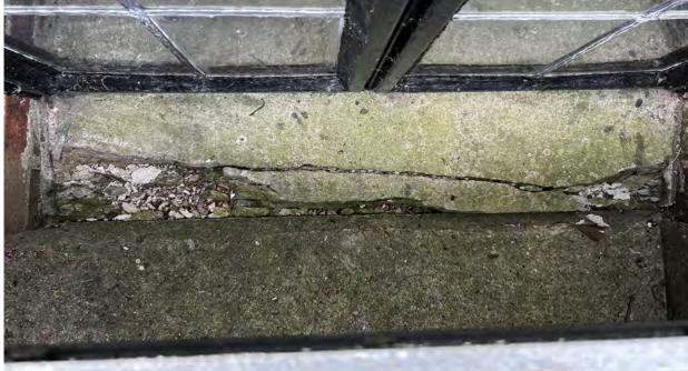
IMAGES 3.1.17 CRACKED CONCRETE SILL
