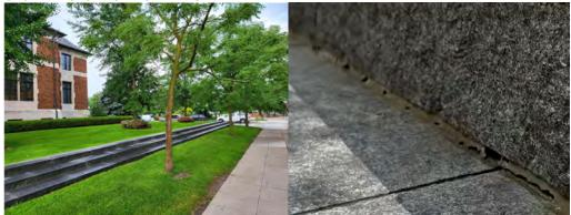
IMAGES 3.1.04 CAULK AT STONE STEPS FAILING
