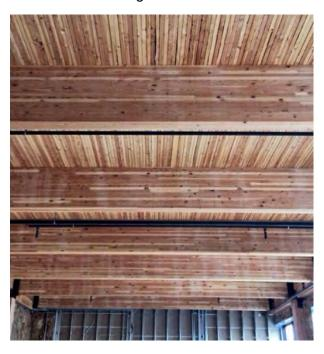
Figure 5.1: NLT and Glulam Girder System
