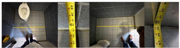
IMAGE 4.2.33 - 1ST FLOOR MENS WATER CLOSET CLEARANCE
