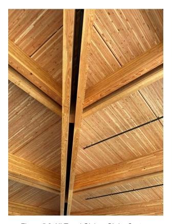
Figure 5.2: NLT and Glulam Girder System
