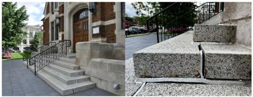
IMAGES 3.1.03 CAULK AT STONE STEPS FAILING
