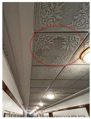
FIGURE 2.3.06 – DUST BUILD-UP ON ACOUSTICAL CEILING TILES IN THE PRIMARY CORRIDORS.
