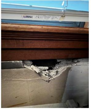
FIGURE 2.3.02 – DAMAGED PLASTER IN THE ASSISTANT CITY MANAGER'S OFFICE.
