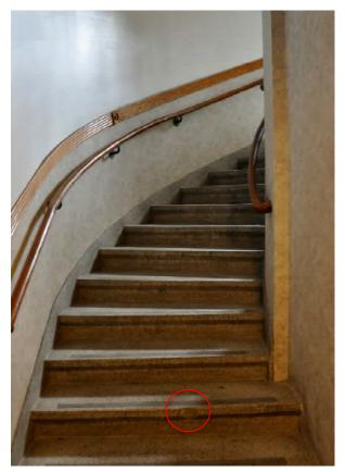
FIGURE 2.3.05 – CHIPPED STAIR NOSING ON TERRAZZO FLOORING.
