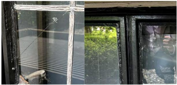
IMAGES 3.1.16 CRACKED WINDOW GLASS AND FRAME COATING
